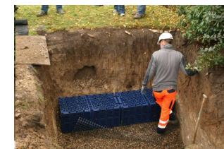
Faskine (plastkassette) nedgraves.
