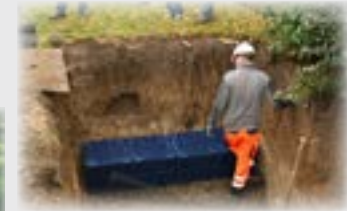
Faskine (plastkassette) nedgraves.
