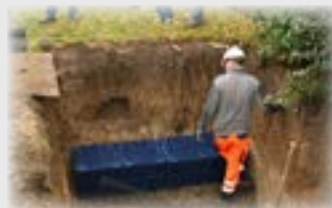
Faskine (plastkassette) nedgraves.
