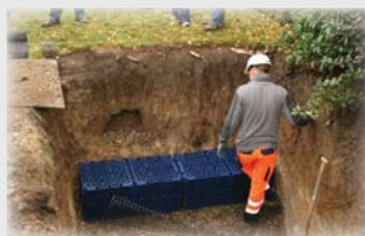
Faskine (plastkassette) nedgraves.
